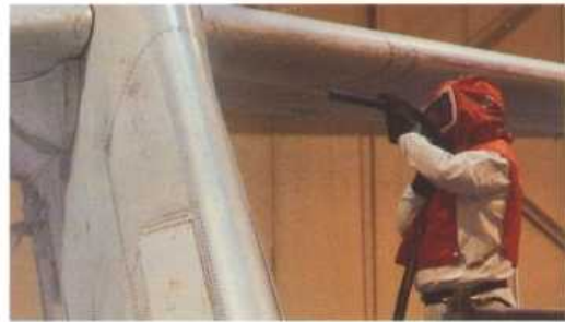
Carefully controlled operating parameters are the keys to success on this DC-9 fuselage.
