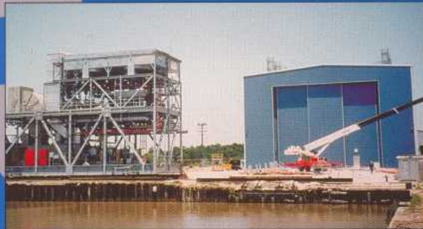
Modified Downdraft Paint Room
