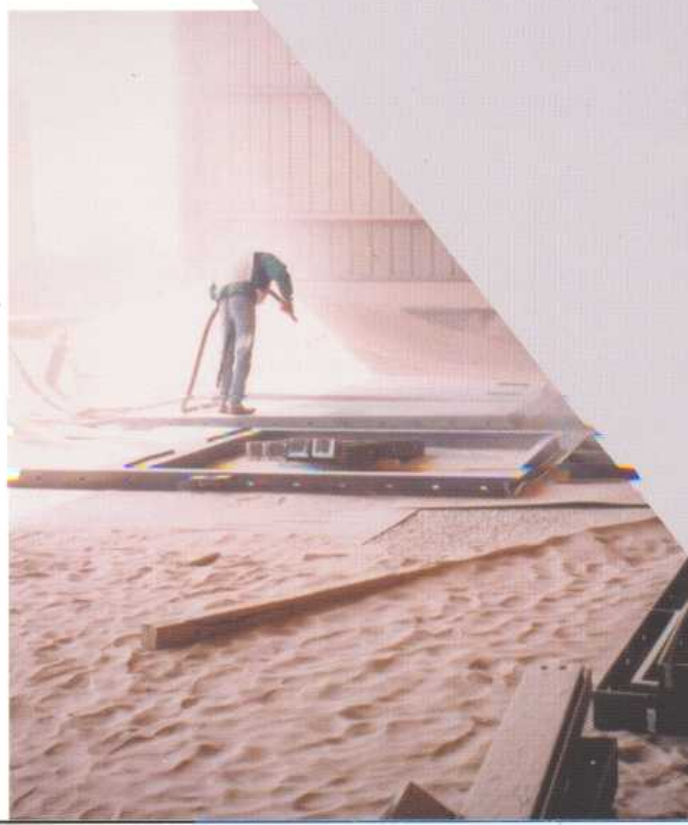
(Before) Traditional sandblast area with poor worker safety and environmental pollution.
